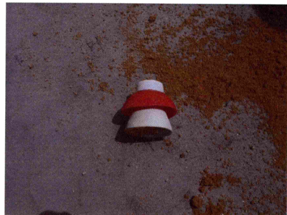
Photograph 20: Detail of the state of one of the protections which ended up inside the bag. There is no perforation of the steel armour through the plastic piece.
